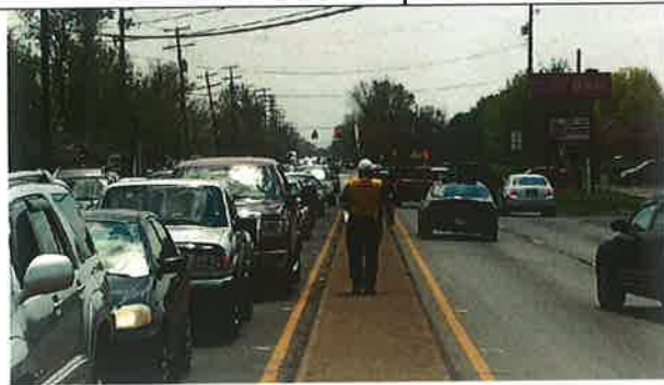
DGK Mike Brunetti working to Measure Up
