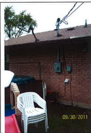
New electrical service box was installed
