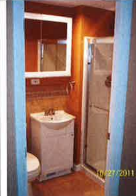
The master bathroom was completely renovated
